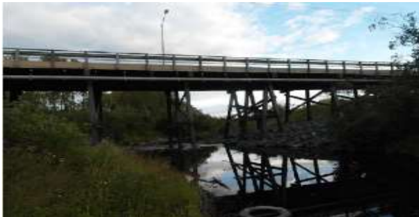
Figure 25 ATIM Road Bridge (BCI=78.2 Good)
